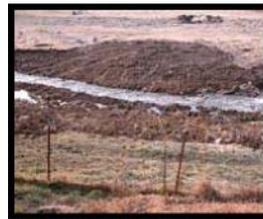
Sites near a stream may require an undisturbed buffer zone. This photo shows a violation of county, state, and federal laws. Get permission before you dig in the creek. Stream culverts require permission from the Army Corps.
