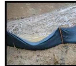
Installing silt fence properly will "pond the water" and let the sediment fall to the ground behind it. You can see from this photo how the weight of water can push silt fence down. This silt fence needs reinforcing.
