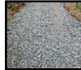
An adequate gravel construction entrance will be 2-3" clean stone. Loose **BIG** stone scrapes mud off tires. Small stone will "pack down" and doesn't work as well. Place stone where vehicles enter the highway.
