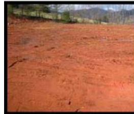
In this photo it is obvious that no attempt to establish ground cover has been made. Ground cover is the best erosion control measure. Ground cover reduces the need for sediment control. Seed and mulch ASAP. It will rain.
