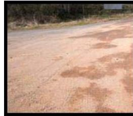
An unsafe condition is created if you allow mud from your site to be tracked onto the public road. You may be held responsible if it causes an accident. An adequate gravel construction entrance can prevent a "mud-slick".
