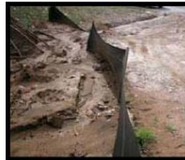
Silt fence that has been installed incorrectly or in an area of concentrated flow will fail. Silt fence works by impounding water (building a pond). "Fence-on-a-stick" will need to be reinforced. Think... "I'm building a pond."
